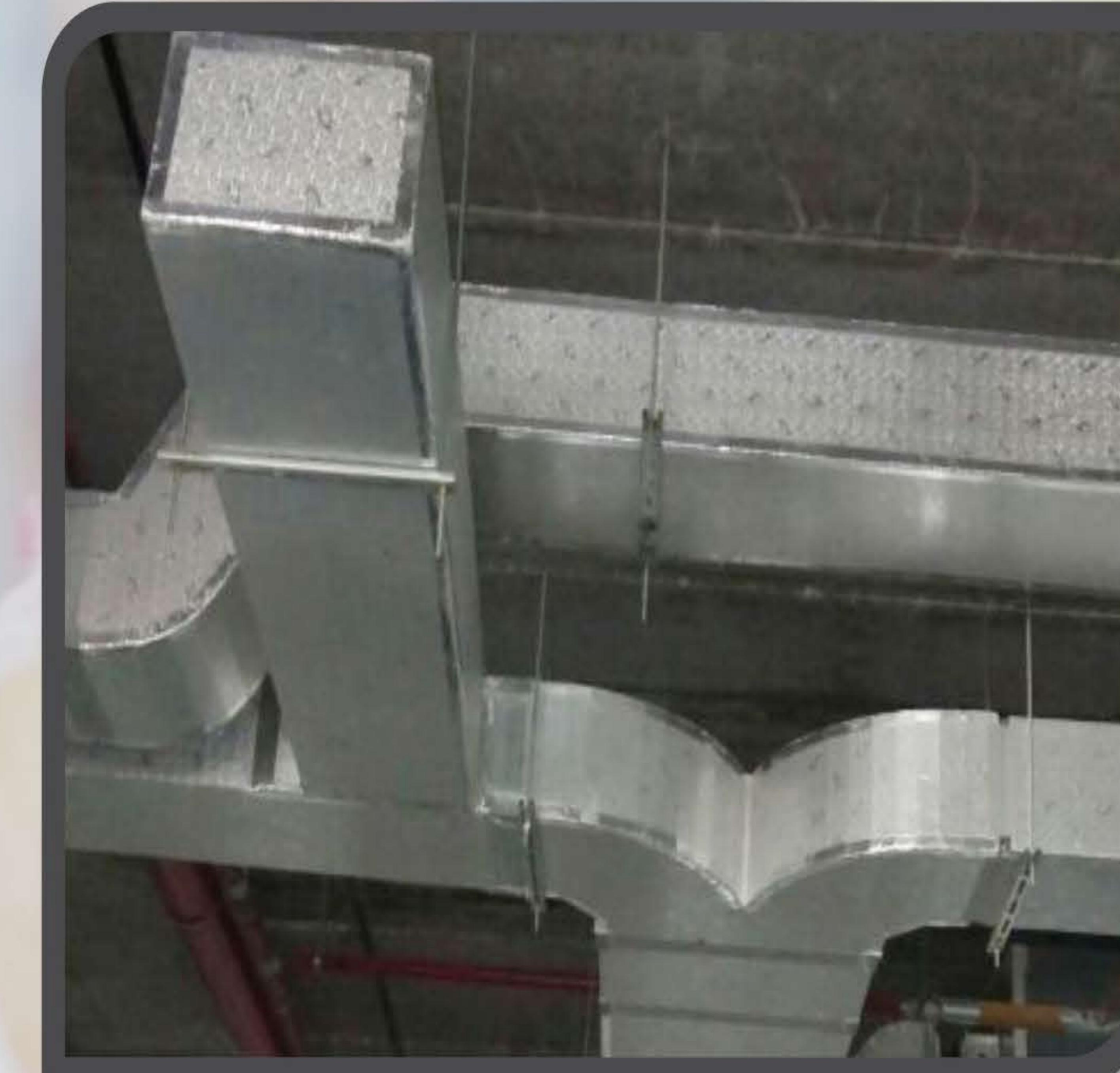
The Ducts are manufactured as per standard EN13403 which are CNC machine cut and are assembled by AIPL employed fabricators. These fabricators are also skilled to carry out entire fabrications as per the standard set by AIPL at site.
